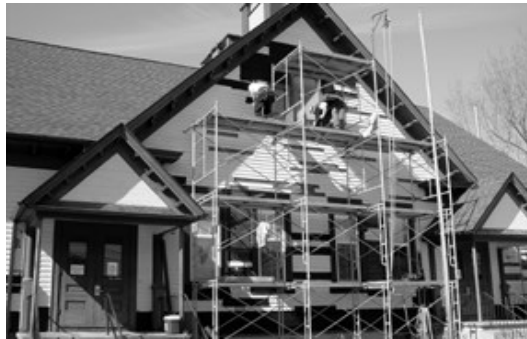
REMOVING DAMAGED CLAPBOARDS
