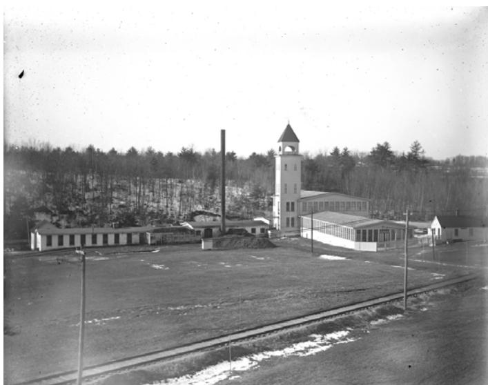
Mohegan Mill with trolley tracks in front of mill Photo taken by photographer, Elmer Harrington Reynolds, early 1900s
